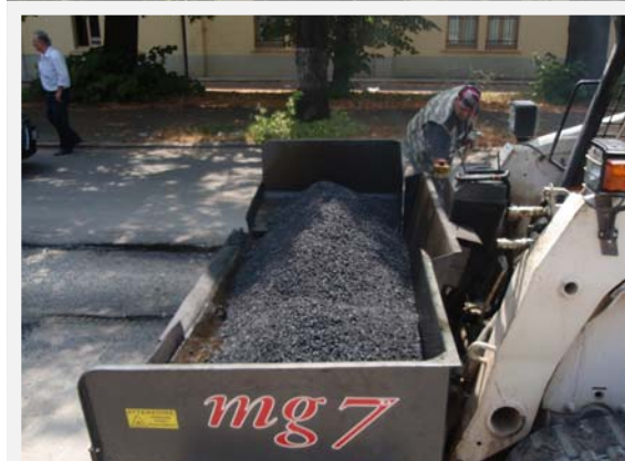
MG7 paving a shoulder.
