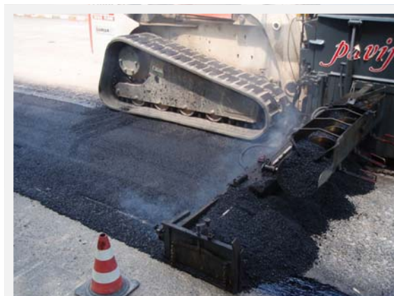
MG7 paving a shoulder.
