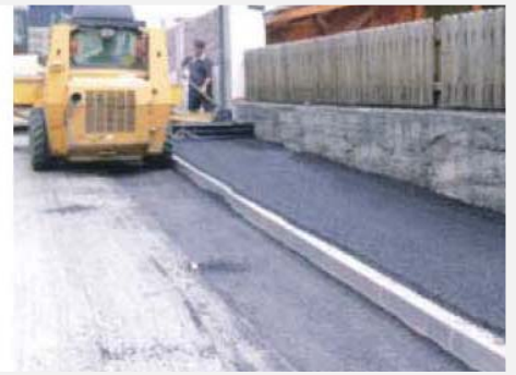
Laying sidewalk around gutter
