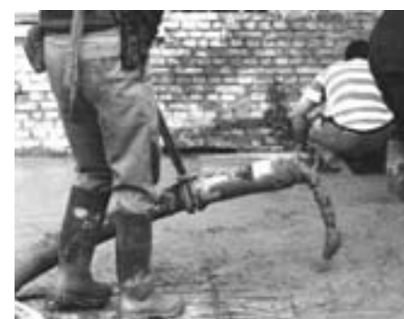
Concrete pumping
